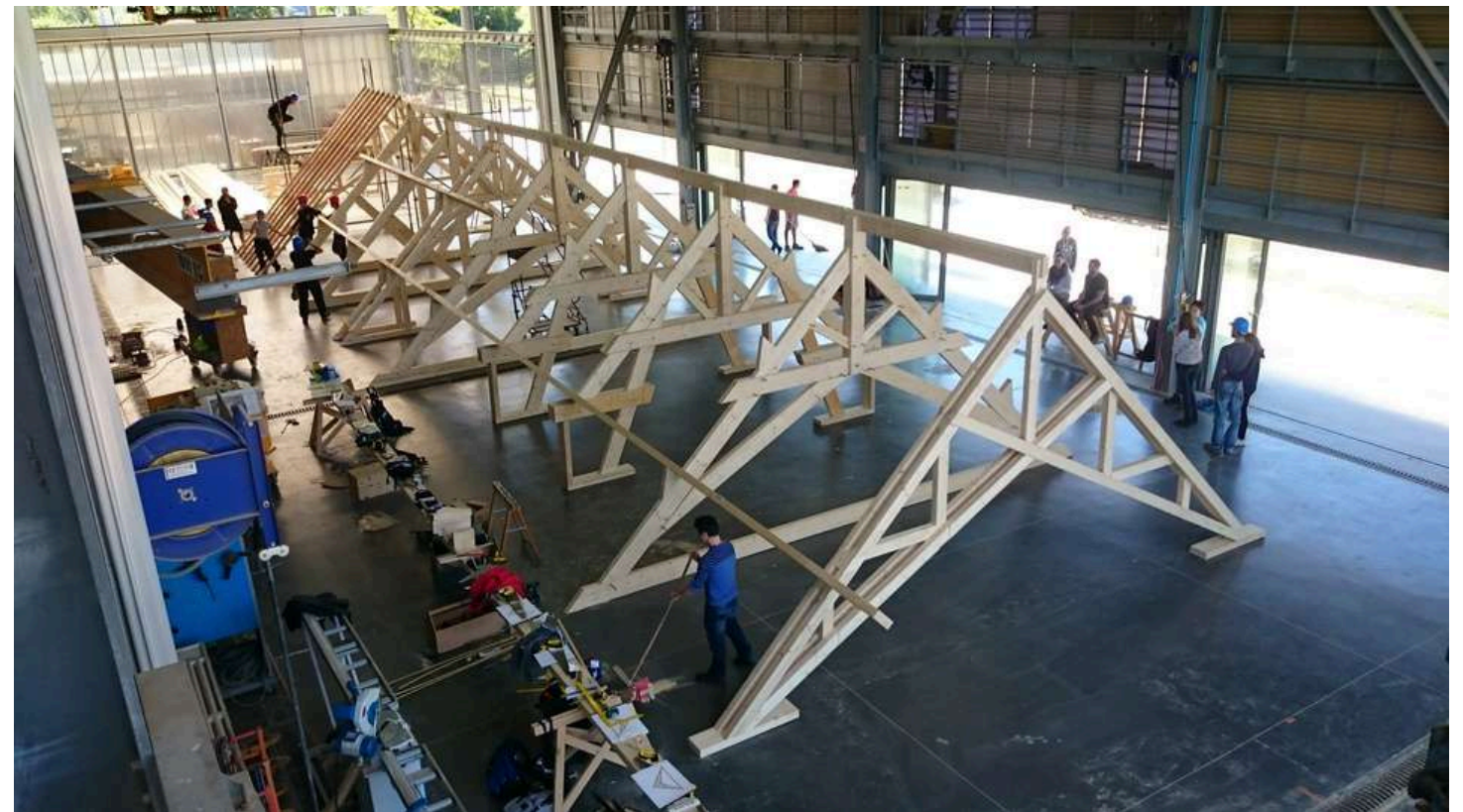
WORKSHOP Constructions de charpente ENSASE - 2018
